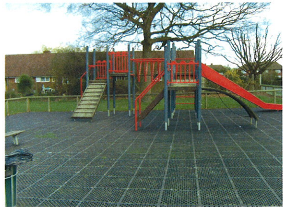
New playing surface at Michael Crescent
