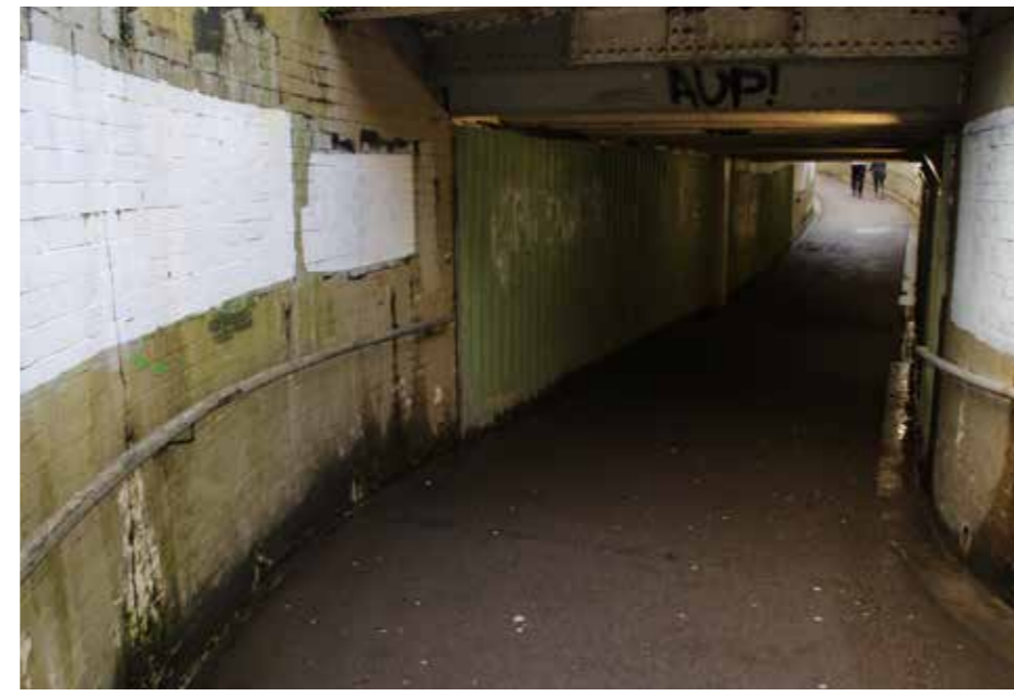
The subway is gloomy with poor visibility and low lighting levels.
